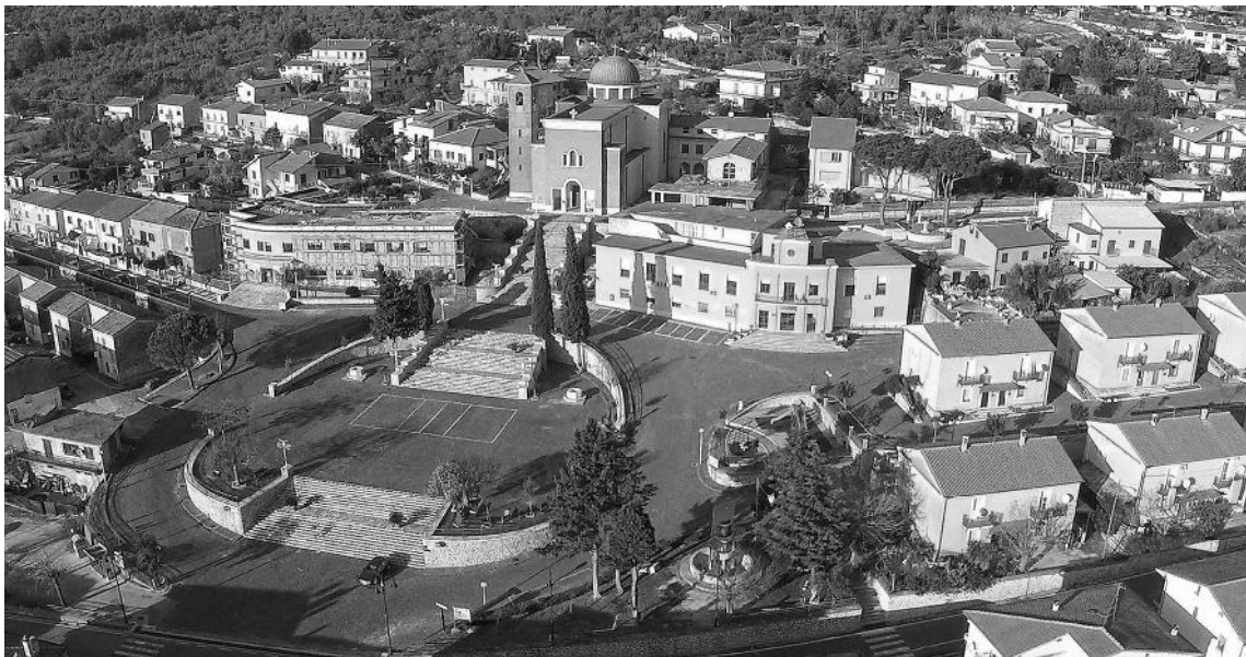
Fig 12 - San Pietro Infine (CE), the new city, built on another site between 1945 and 1950.
