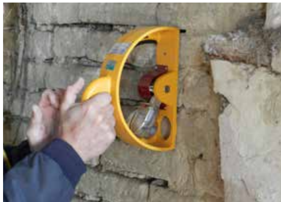
Figure 9. On site rebound test (credits Manuela Mattone)
